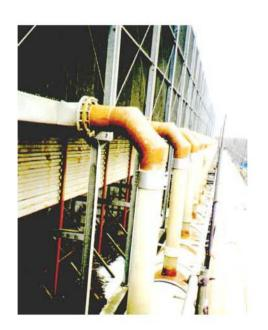
126 couplings were installed in two nine hour nightshifts without disruption or shutdown to the lines.
