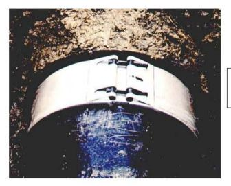
Axiflex HC Couplings were retro-fitted to these new GRP pipes to allow thermal and axial movement.
