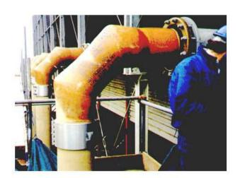
This large diameter water main was repaired in minutes without shutting down the line.
