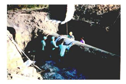
Teekay Axiflex or Axilock Couplings can be used for "cut in" repairs, where a new piece of pipe is inserted into an existing pipeline.
