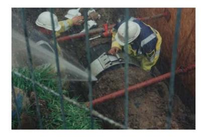
The leak is located and the area around the main is excavated. In this case, the 27" steel trunk main has a 1"hole.
