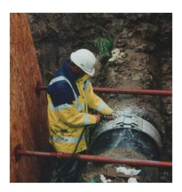
With the Repair Coupling in position, centred over the hole, the screws are quickly tightened. This can be done with a combination of speed brace and torque wrench. Here the fitter is using an air gun with an allen key attachment. The tightening is done in stages, going evenly from one screw to the other.
