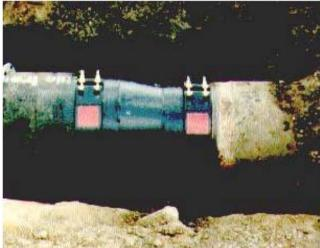
Stepped or Reducing Couplings can be used where the new pipe has an O.D. different from the old one.
