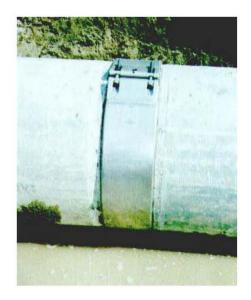
Leaking joints can be replaced in situ without moving the existing pipework.
