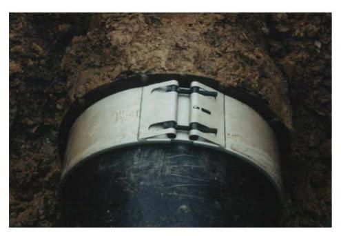
The tightening is completed by torque wrench to the value stated on the coupling label. This figure may be increased, depending on the pipe material and its surface condition.
